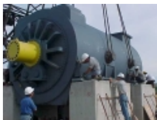
Generator Installation
