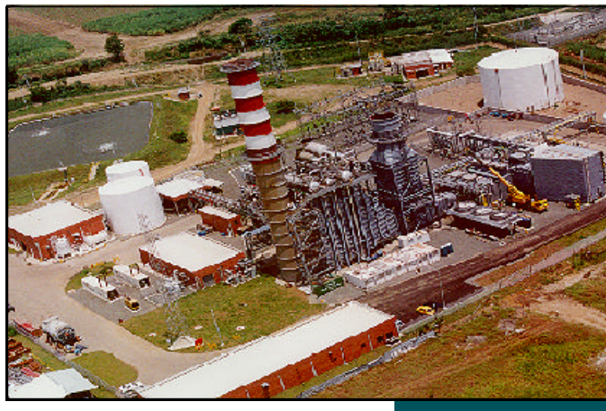
240 MW Termovalle I oil/gas-fired, combined-cycle plant utilizing 501F technology
