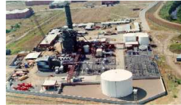
240 MW Termovalle Power Project Cali, Colombia
