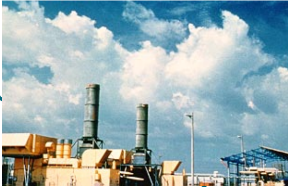
100 MW Mamonal Power Plant Cartagena, Colombia
